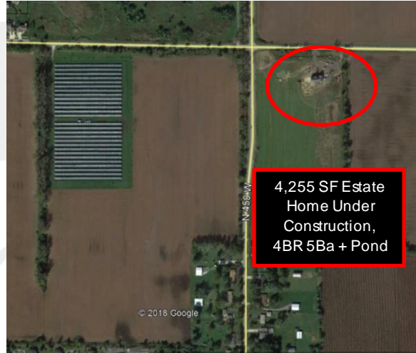
Portage Solar Farm, IN October 2016
